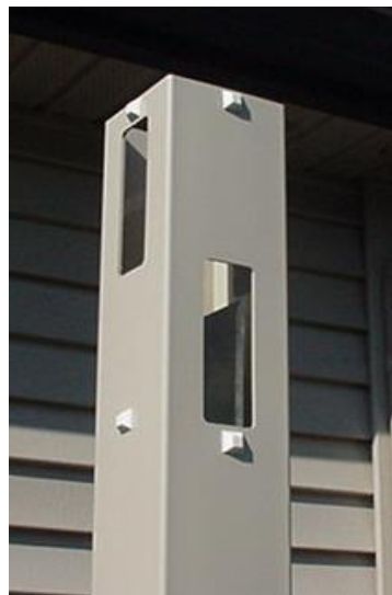
Adhesive spacers align sleeves with posts
